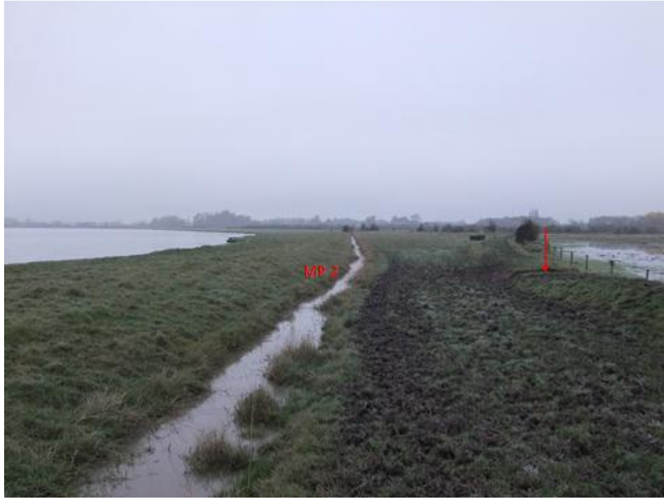
Figure 3.9 Monitoring Point 2 at high tide, 15 th November 2012 (arrow marks the breach in the old sea wall).
