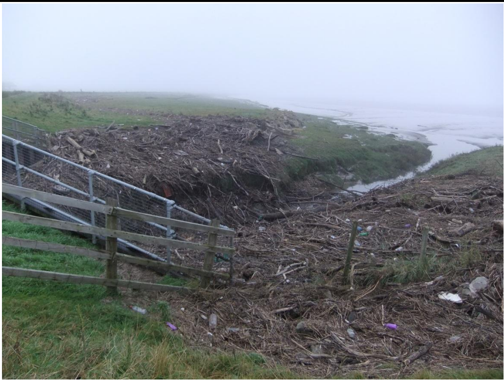
Figure 5.1 Hock Ditch outfall, 21 st October 2012 with wrack from recent high tides
