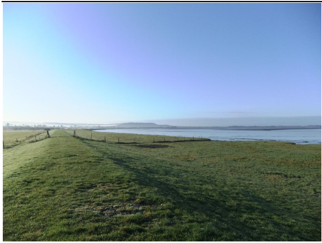
Figure 2.1 The Environment Agency's embankment on Saul Warth is kept clear to aid inspection and discourage mammals and vegetation from weakening the defences, 25 th February 2012
