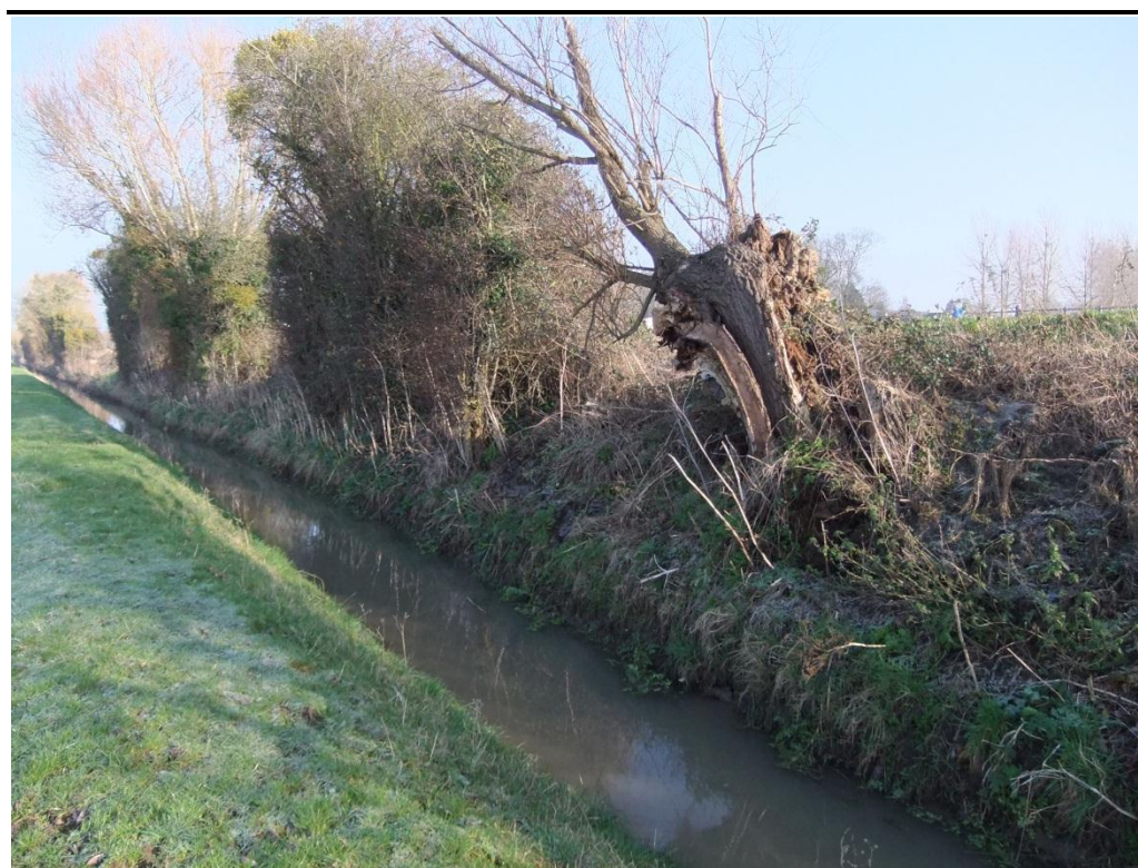
Figure 2.3 The primary drainage channel beside the western canal bank at Frampton, 13 th January 2013
