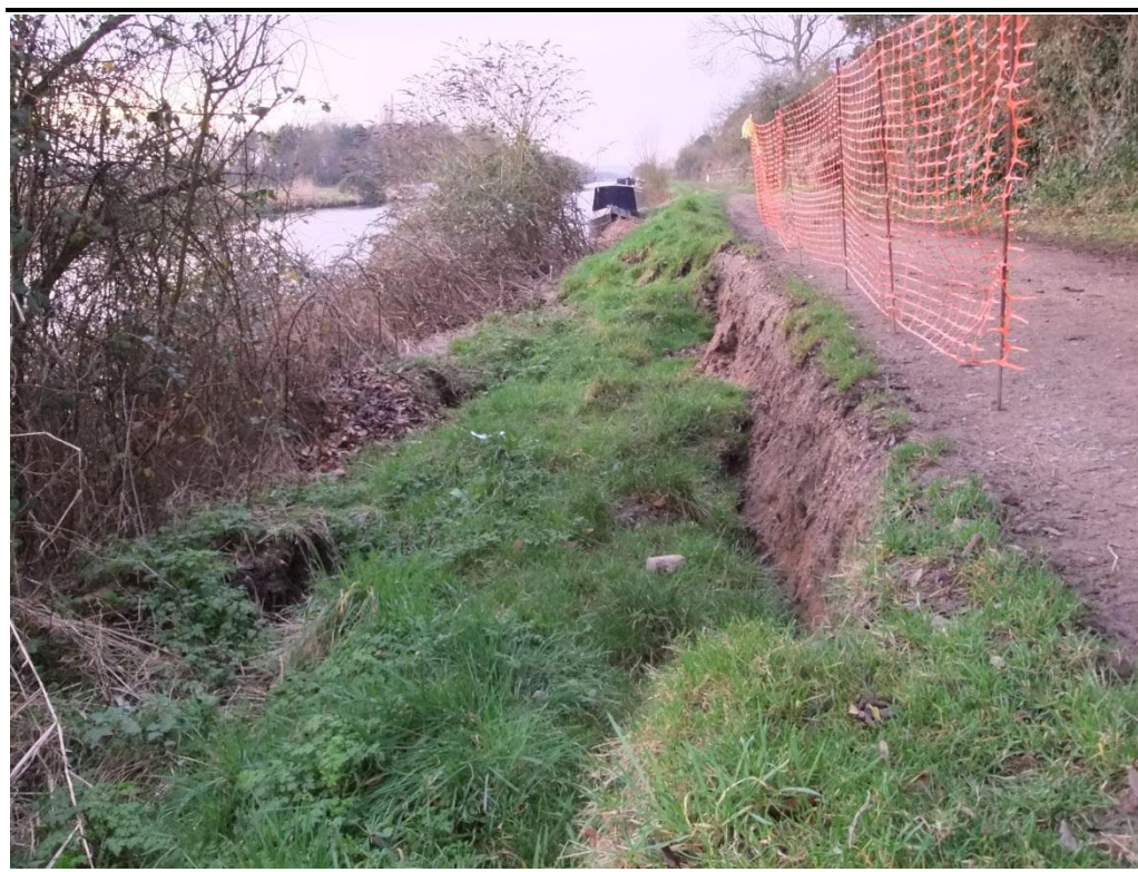
Figure 6.1 Canal bank slippage near Saul Lodge, Fretherne, 8 th January 2013
