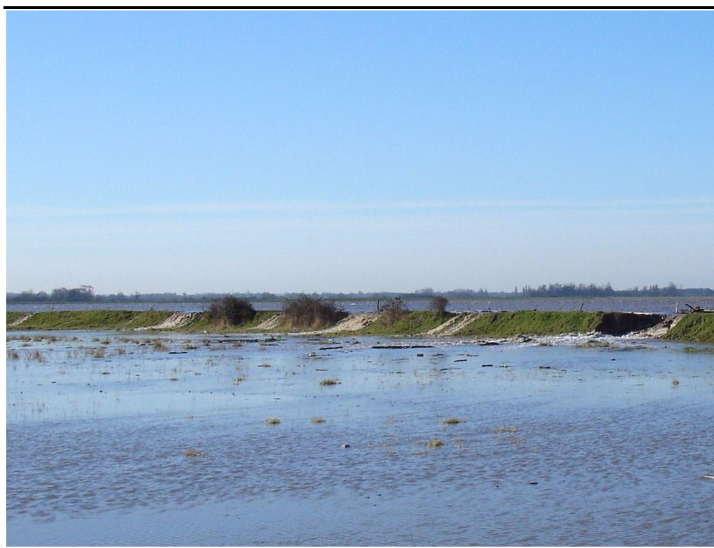
Figure 7.2 Tide topping and breaching the abandoned sea wall on Frampton Warth, 2 nd March 2006
