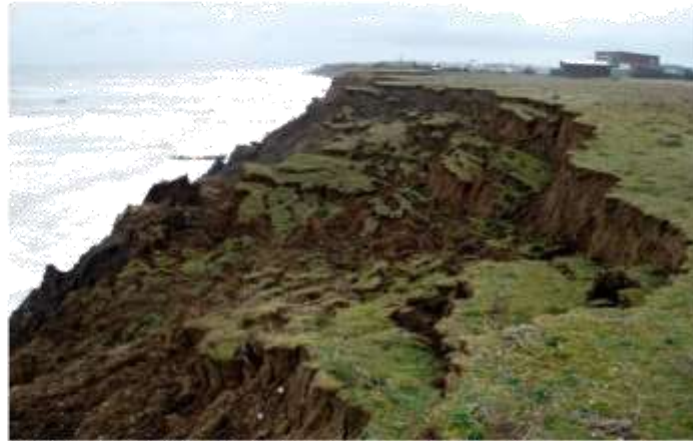
Eroding cliff line: 48 km
